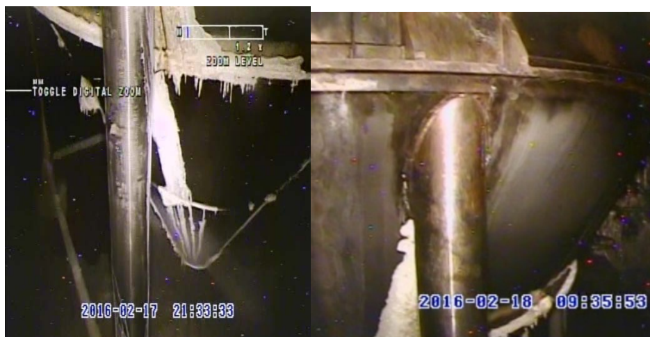
Fig. 4. Figure on the left shows visible salt deposits on the lagging of the evaporator vessel. Figure on the right shows one of the location where the leak is coming out of the vessel lagging where the leg penetrates thru.
